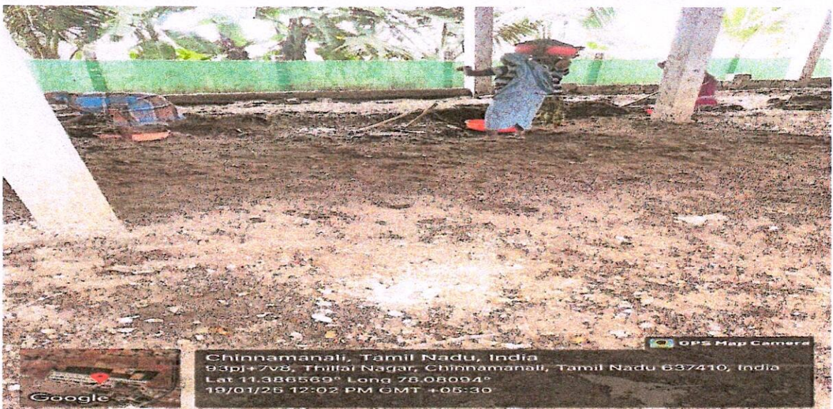
Visibility of impermeable layer after the collection of manure
