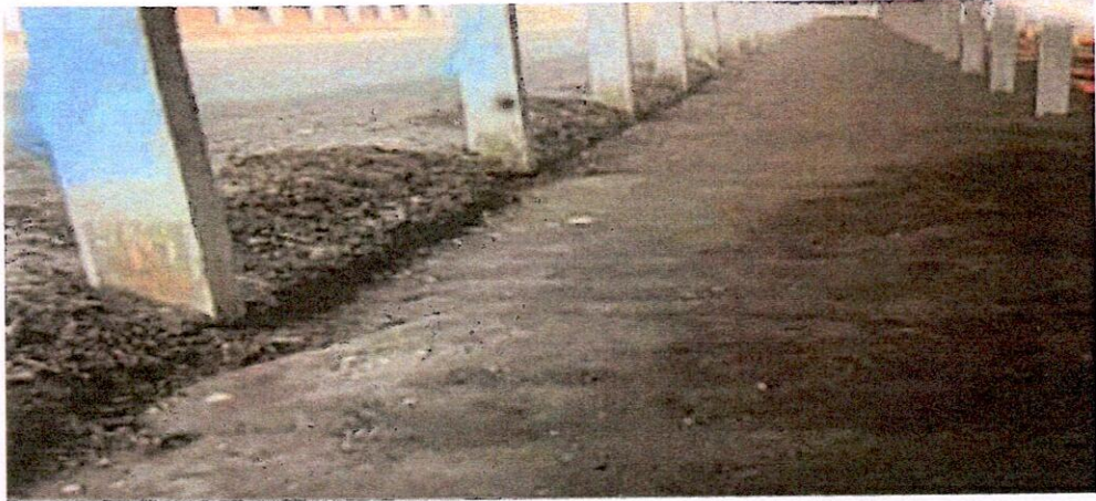
AFTER COMPLETION TO IMPERMEABLE LAYER
