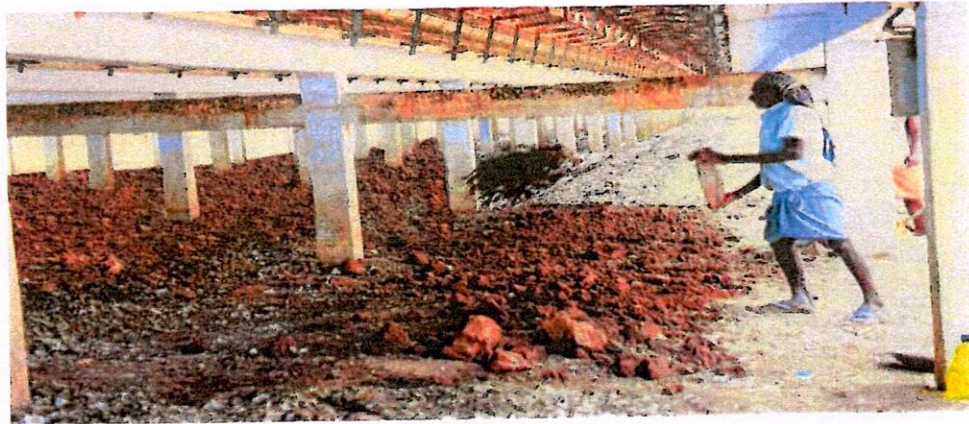
Spreading of clay
